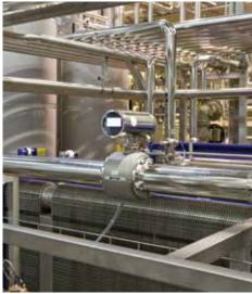
FLOW MEASUREMENT OF DEMINERALIZED WATER
